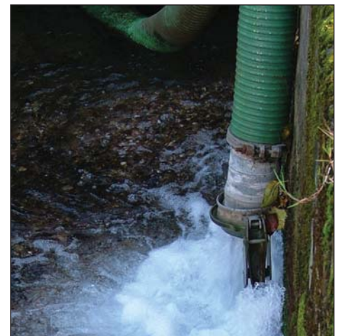
Pumping water discharge
