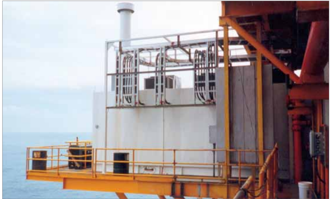
An offshore 800-kVA at 480 V VSD module for the Gulf of Mexico.
