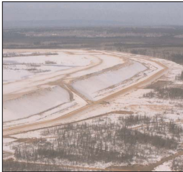
Site characterization of the open pit mine
