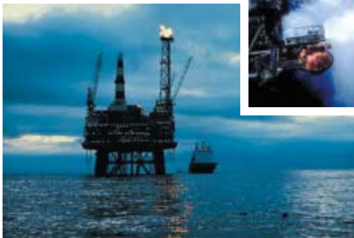
^ Flaring during well testing of a discovery well in the Gulf of Mexico ( inset ). Worldwide, the industry flares or vents 2 Tcf [57 billion m 3 ] of gas per year. GTL technology may offer ways to bring to market gas that is currently flared or vented. (Photographs courtesy of Energy Data Solutions, LLC, www.ocsbbs.com )
