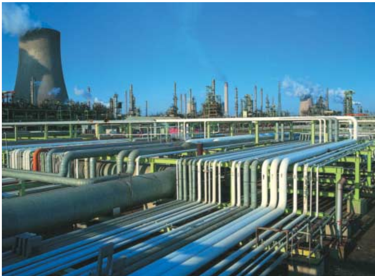
^ Sasol Synthetic Fuels, Secunda, South Africa. Sasol operates two such plants, applying gas-to-liquid (GTL) technology to convert coal-derived natural gas to liquid fuels. (Photograph copyright of Sasol Limited.)
