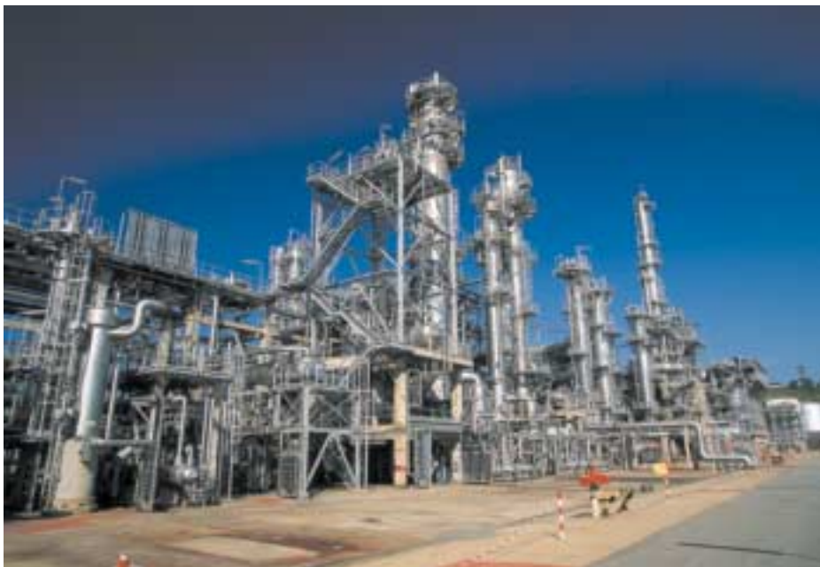
^ Shell GTL plant in Bintulu, Malaysia, in operation since 1993. Using a patented Shell process, the Bintulu plant converts natural gas piped in from Sarawak to 12,500 B/D [1990 m 3 /d] of clean diesel, kerosene and naphtha. (Photograph courtesy of Shell Chemicals Singapore.)
