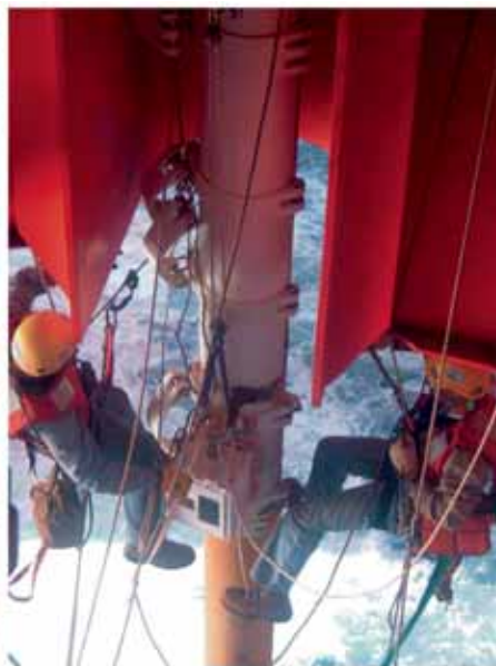
Rope Access Deployment
