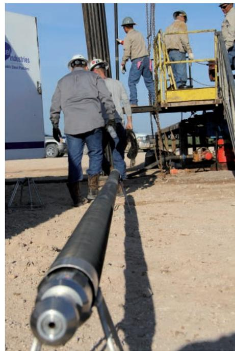
*The Saltel expandable steel patch enabled the operator to safely and successfully fracture the well despite a derated external casing packer valve.*
