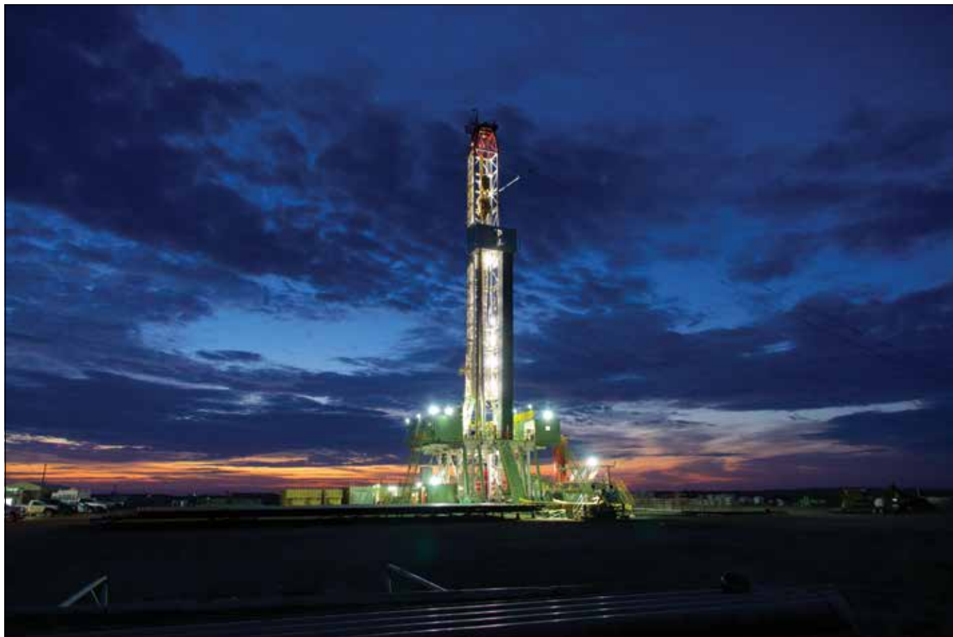
Precision Drilling's Rig 580, a Super Triple 1500 series rig, works in Oklahoma. The company is using similar-design rigs, deployed on turnkey jobs in Louisiana, to deploy the new remote directional drilling service. Turnkey jobs are serving as a proving ground for the service.
