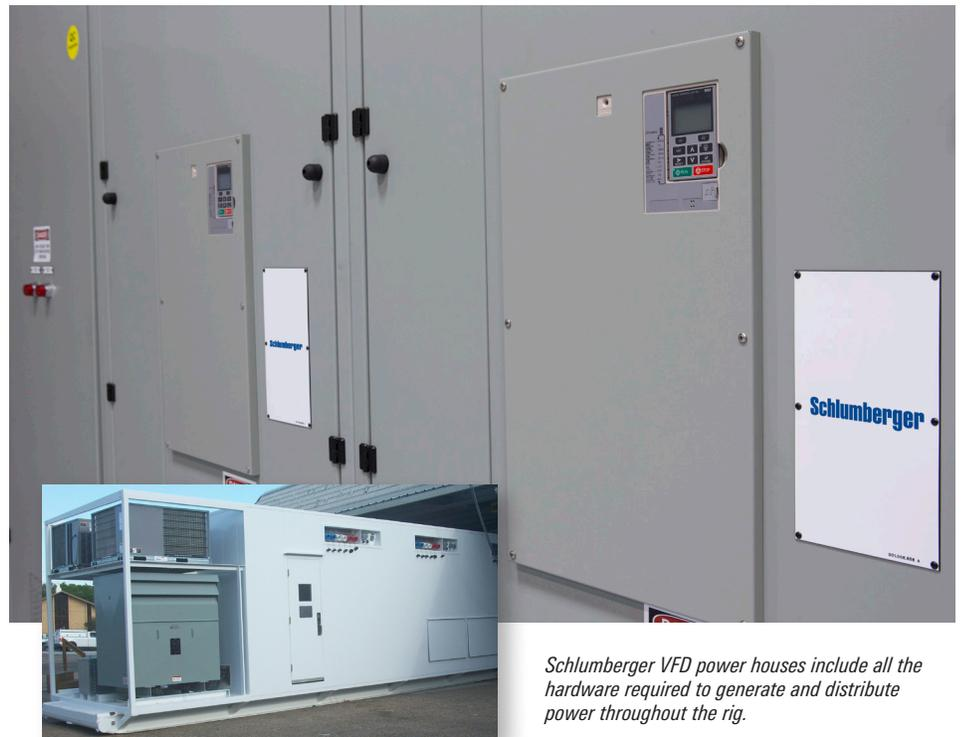
*Schlumberger VFD power houses include all the hardware required to generate and distribute power throughout the rig.*
