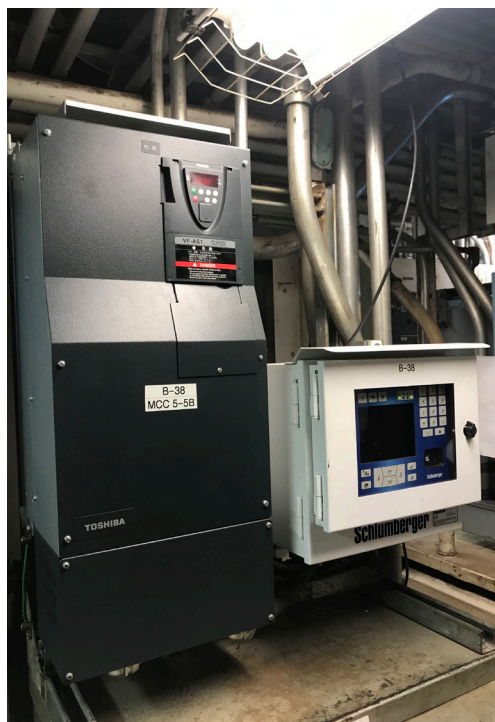
Small installation footprint of low-voltage variable speed drives with Instruct control units.
