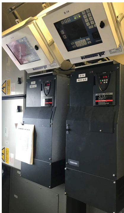
Small installation footprint of low-voltage variable speed drives with Instruct control units.
