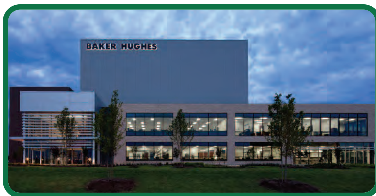
At the Artificial Lift Technology and Research Center in Claremore, Okla., engineers test alternative intervention methods, conduct system integration testing and work to increase ESP system reliability in harsh environments. (Photo courtesy of Baker Hughes)
