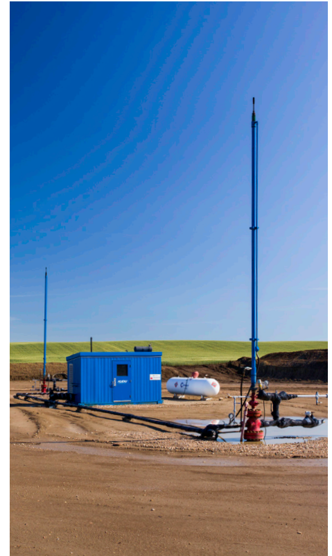
KUDU HPU and power unit installation.
