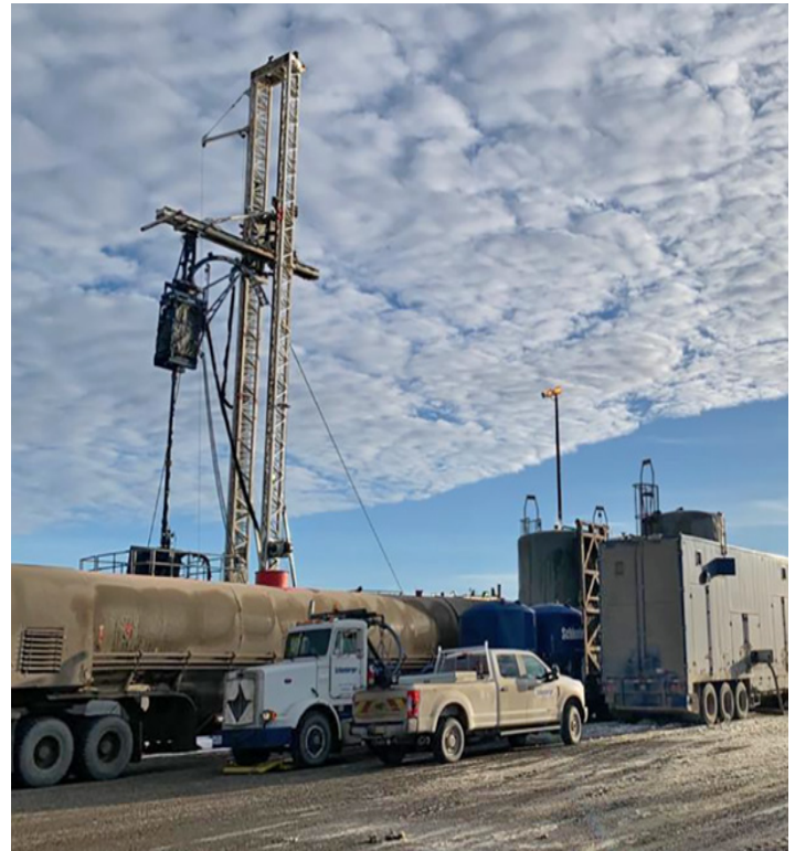
The operator managed SCP in a challenging field with a CT squeeze of CemFIT Heal system, which has high flexibility under stress and an ability to heal any cracks that form.
