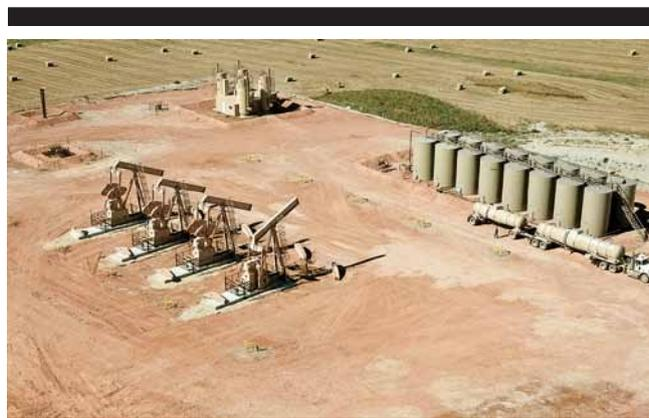
**Fig. 3.** Producing wells on one of the 40 ECO-Pad drilling locations that Continental Resources intends to have in operation by the end of this year. Continental credits the technique with reducing costs as much as 10% per well. Courtesy of Continental Resources Inc.
