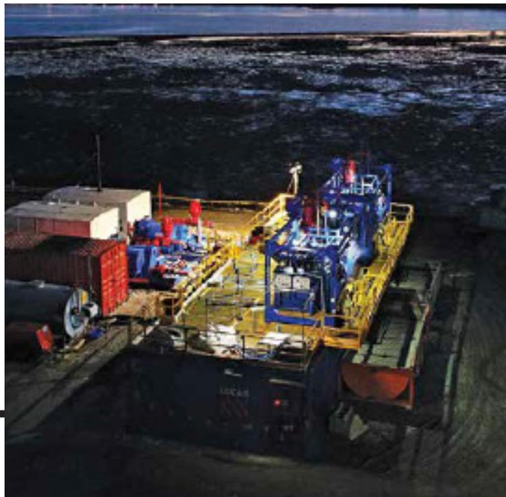
HDD crossing of the Tauranga Harbor, New Zealand, for the installation of a new sewer pipeline.
