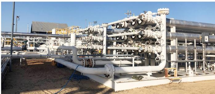
For the final stage of processing, the treatment plant uses two trains, each containing 84 membranes arranged in three banks.
