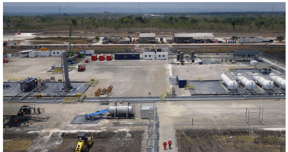
Production was initiated in less than 5 months with a customized facility design of the Veloceti early production system.
