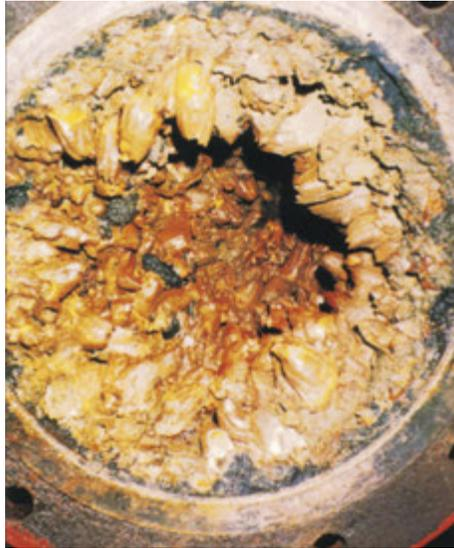
*An example of a severely fouled pipe from a system without a BFCC system.*
