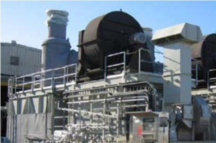
NATCO CHF controlled-heat flux heater with 1,000-degF process outlet temperature capability.
