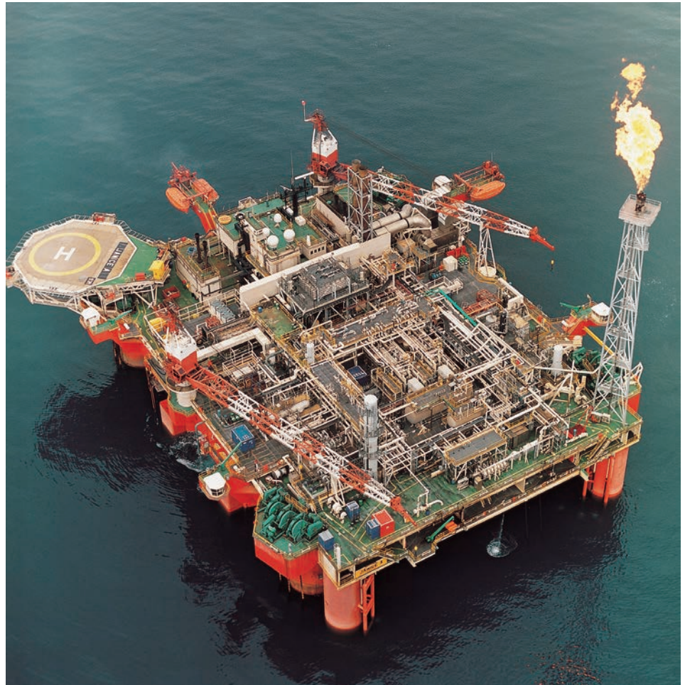
First sulfate removal system installed on floating production unit.
