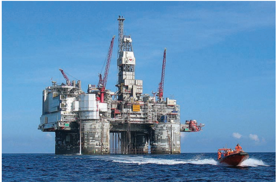
Sulfate removal system installed on Equinor Heidrun platform.
