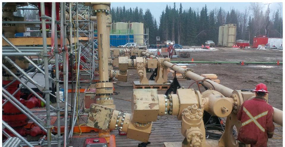
*The Monoline technology used a series of 5½-in high-pressure pipe segments joined together with 90° elbows and swivel flanges, eliminating leak paths and reducing safety hazards. A single modular manifold connected to as many as nine wells on one pad.*
