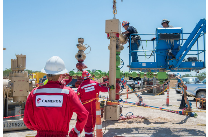
A four-person crew installed the preassembled system in 2.5–3 hours per well.
