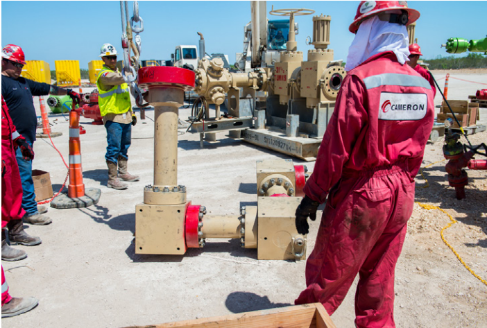
Cameron technicians assemble the Monoline technology at the wellsite.
