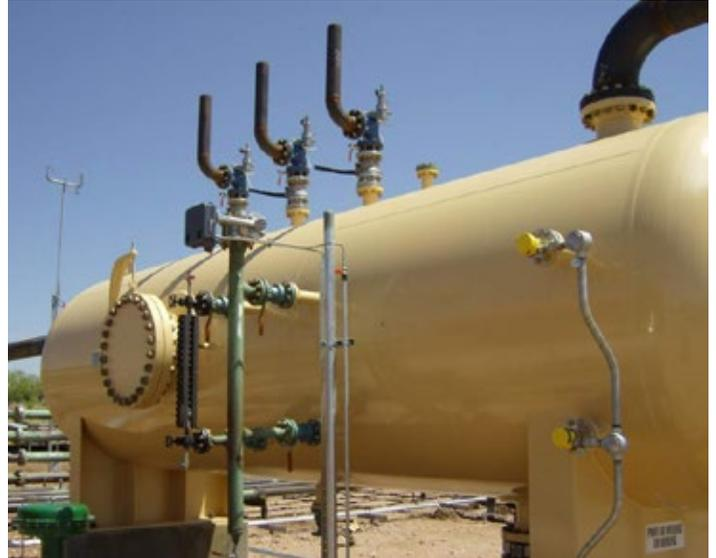
*Valves used during separation must be designed to last since the process fluids may still be corrosive and contain abrasives and chemicals.*
