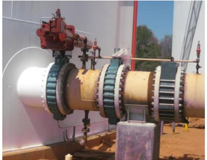
*Inlet valves on a tank need to be able to withstand, and close against, high pressures routinely as it stores the various liquids, gases, and produced water.*
