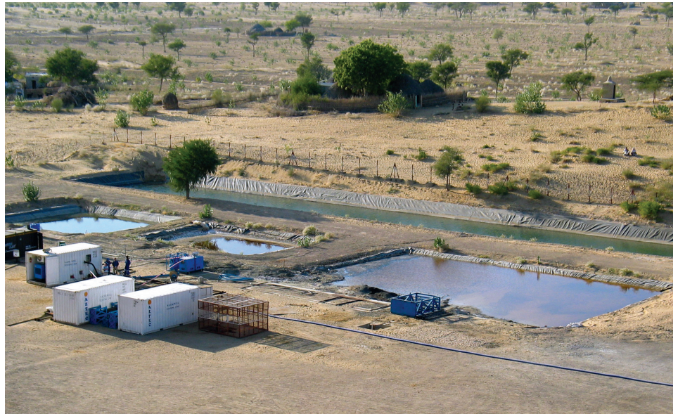
Test pumping site.
