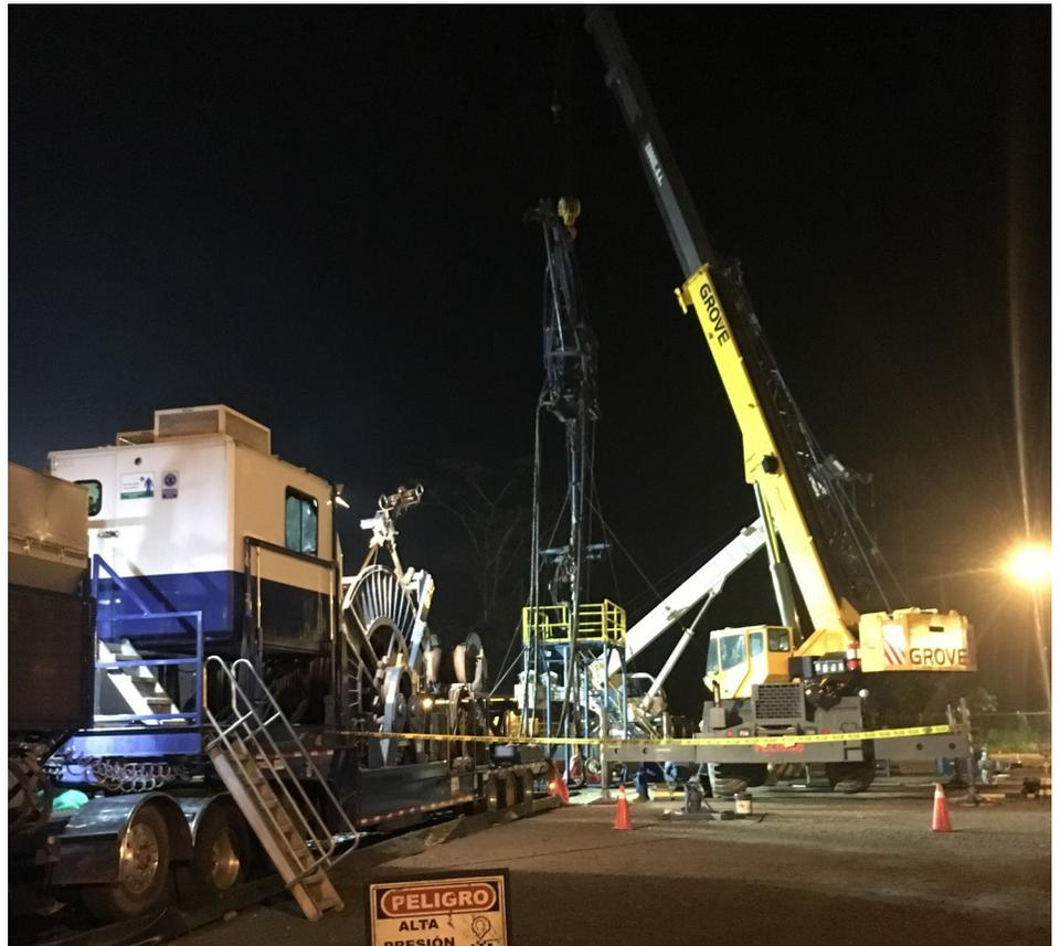
*The ZEiTECS Shuttle system enabled rapid ESP replacement without a workover rig, reducing costs and eliminating more than 5 days of deferred production.*
