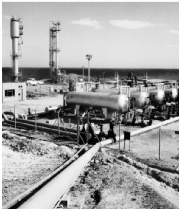
Figure 16.7: Das Island separators and hydrogen sulfide plant seen from the base of the flow tanks
