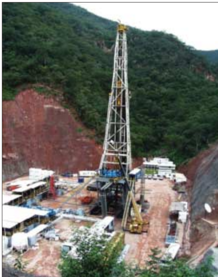
▲ Petrobras remote location drilling. Petrobras is drilling multiple well templates in the San Antonio field in southern Bolivia.
