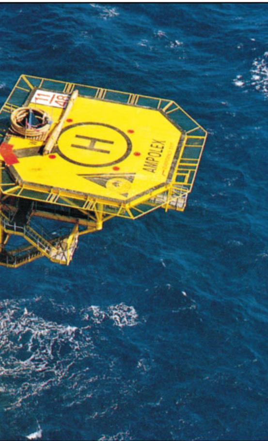
□ Wandoo A monopod, in 52 m [170 ft] of water, offshore Western Australia. All Wandoo production wells have been drilled from this platform. Work is underway to develop the Wandoo B production platform to accommodate eight horizontal wells. (Courtesy of Ampolex Limited.)
